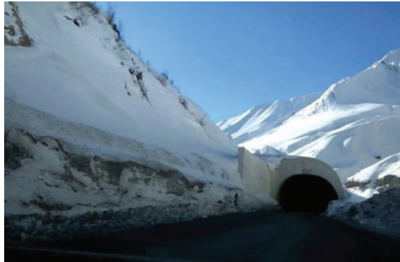
Current road: narrow, unlit tunnels
